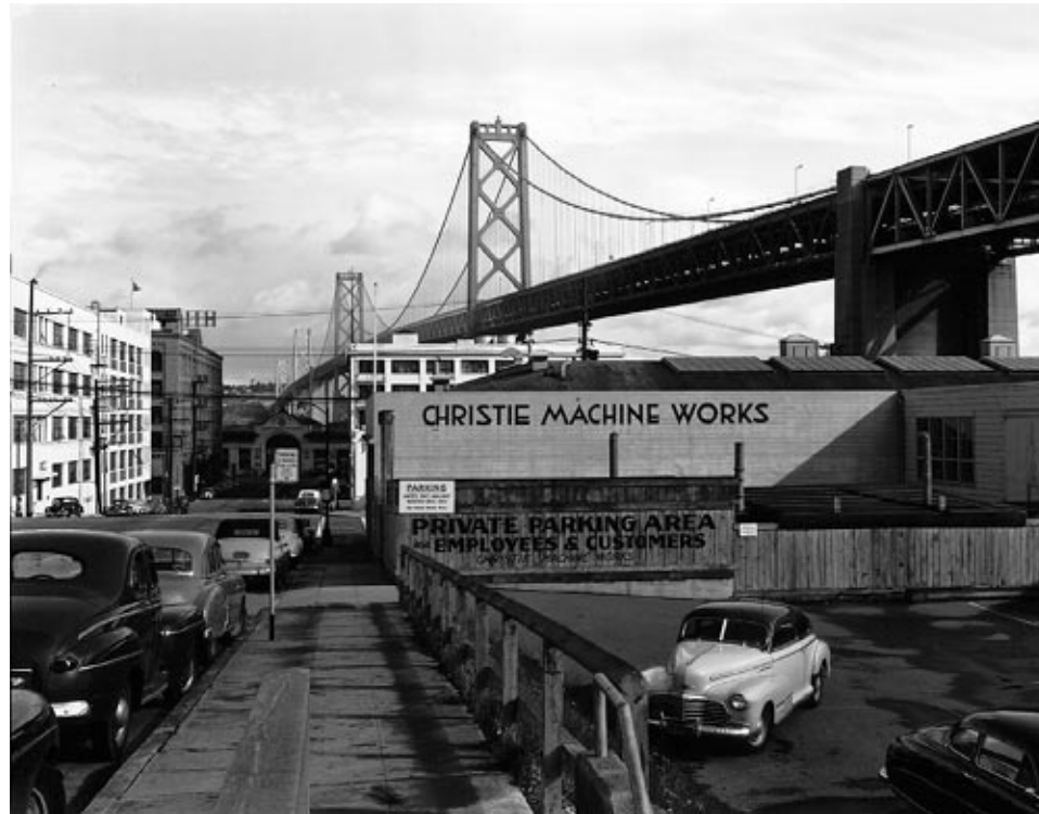
Nr. 501105. San Francisco-Oakland Bay Bridge. 1950
